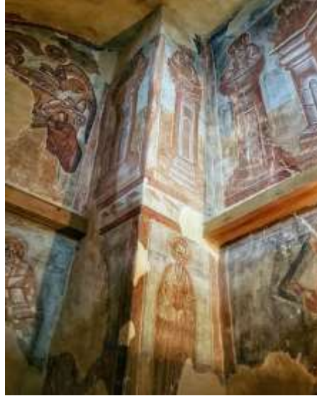
9. View of the corner paintings of the south and west walls of the chapel. Church of the Transfiguration on Novgorod's Ilyina Street
